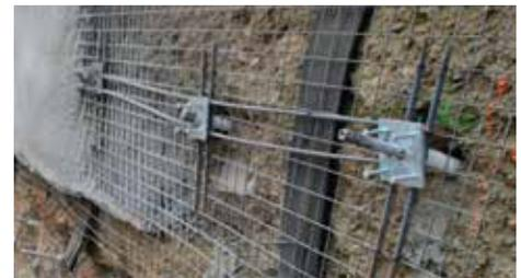
sub-surface conditions. Nucor Skyline provided R38 hollow bar anchors, totaling over 4,200 galvanized, 3-meter bars. The design load of the hollow bar piles was 13.6 kips and was tested to 27.2 kips.
